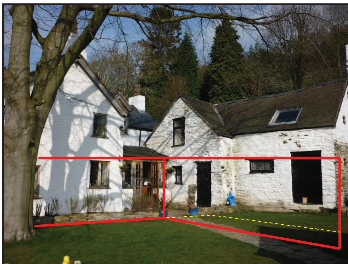
Photo 2 – Tree protective fencing location & ground protection boards to be laid
