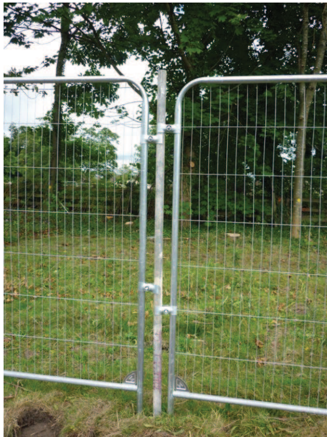
Example of Tree Protective Fencing Specification
