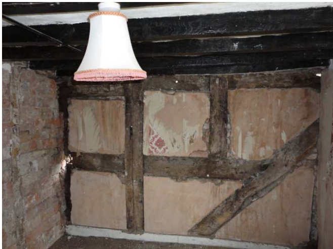
View east towards the timber framed gable end wall.
