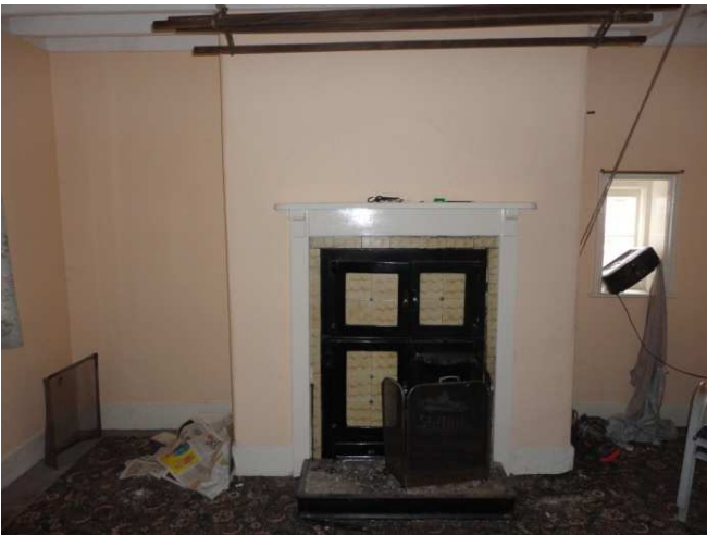
South wall of Living Room showing Buckley brick steps leading up to the Hall, timber staircase leading up to the rear bedroom to be retained and cupboard under the stairs to be retained. Painted beamed ceiling to be retained.
