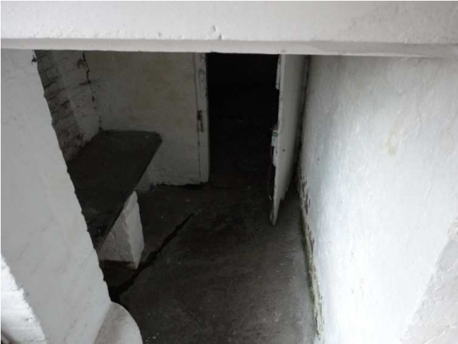
Slate slab in small basement room
