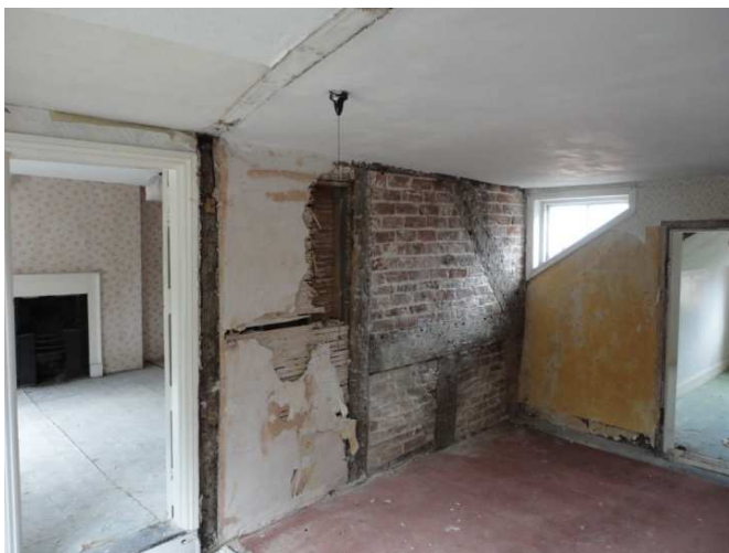
View north west on the landing showing revealed timber frame partition and triangular window which are proposed to be incorporated into the new family bathroom. Existing ceiling to be retained/repaired.
