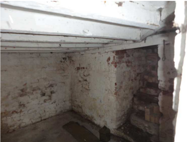
Limewashed walls and floor joists
