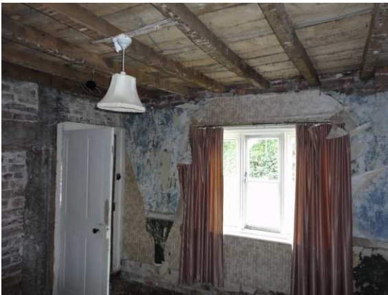
Window in Reception Room
