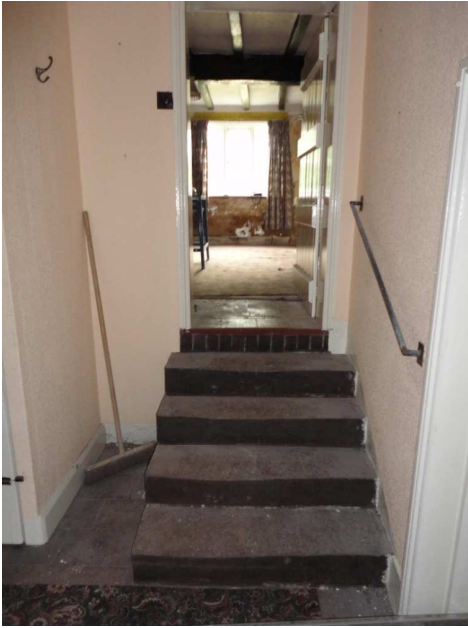
Four Buckley brick steps leading into Hall to be retained.
