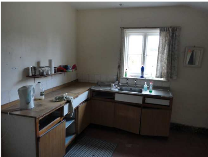
Kitchen, plastered walls and ceiling to be retained.
