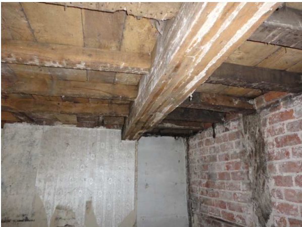
Spine beam and joists in large Reception room.
