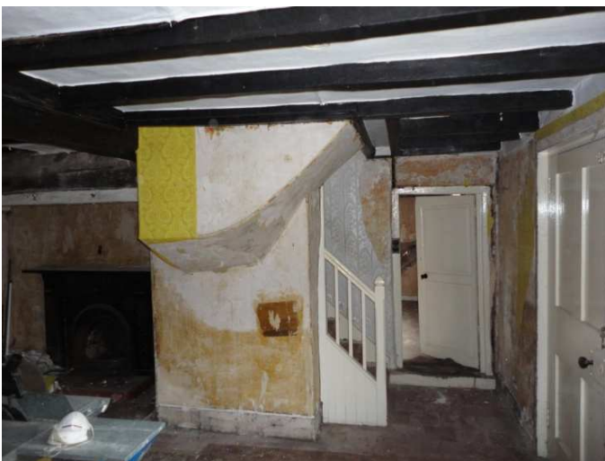
View east within the Hall showing relationship of the staircase to the inglenook fireplace, showing the two-paneled door leading into the smaller reception room, and the four paneled front door. Beamed and plastered ceiling to remain in-situ.
