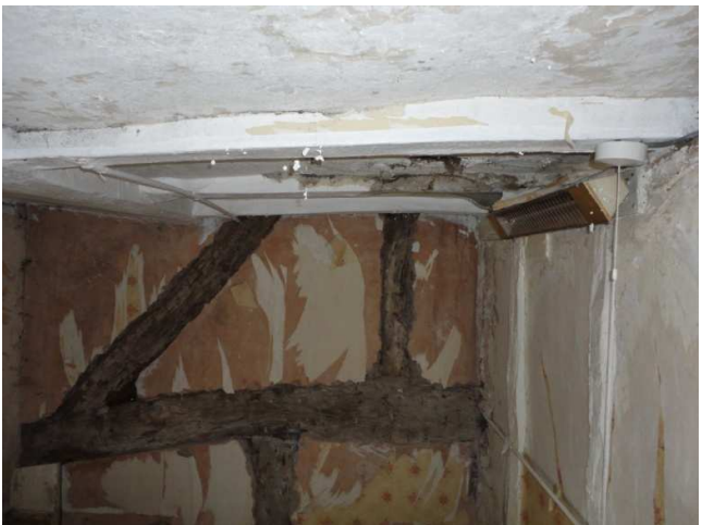
Exposed timber frame of gable end wall in the small bedroom and the bathroom attached to it.
