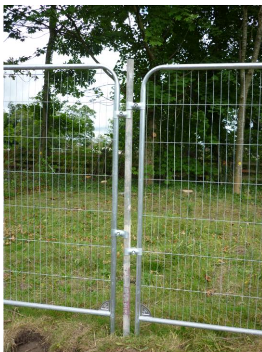
Example of Tree Protective Fencing Specification
