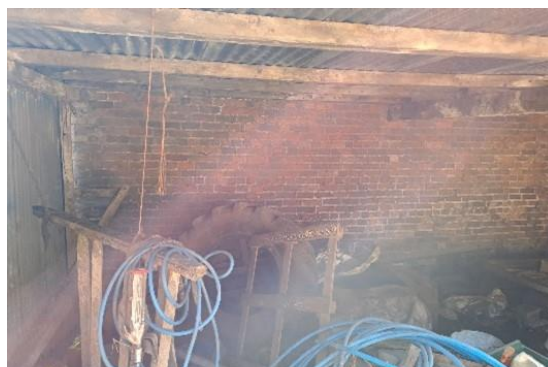
Figure 16: Building B11 internal
