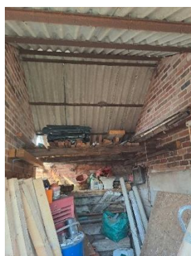
Figure 6: Building B3 Internal
