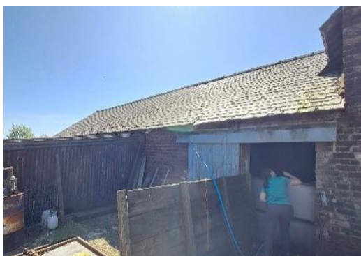
Figure 15: Building B11 external
