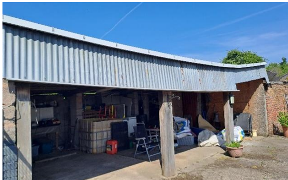
Figure 3: Building B2 External
