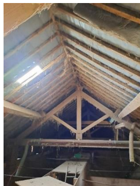
Figure 14: Building B10 Internal
