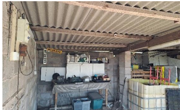
Figure 4: Building B2 Internal
