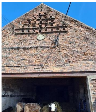
Figure 13: Building B10 External
