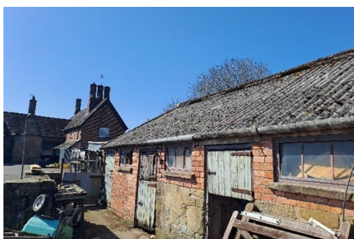
Figure 5: Building B3 External
