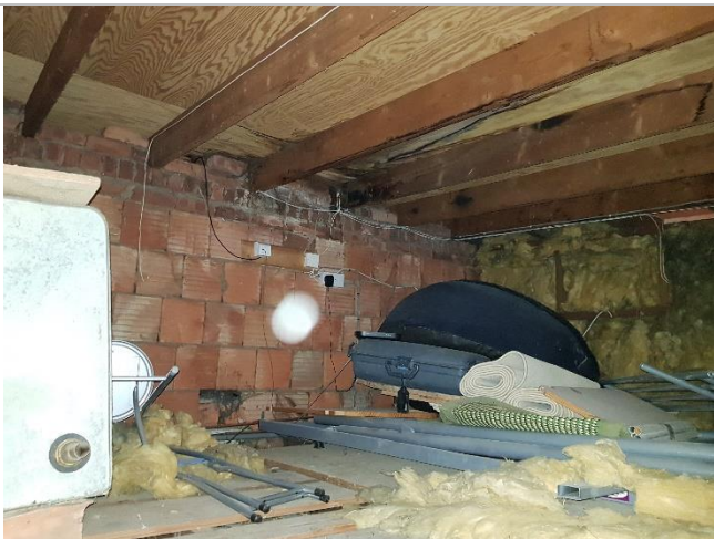
Interior of roof void.
