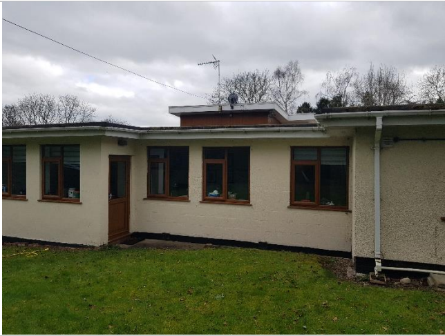
Area of the house to be extended (NW).
