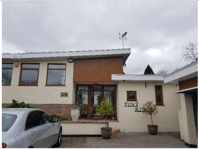
Small roof void above entrance.
