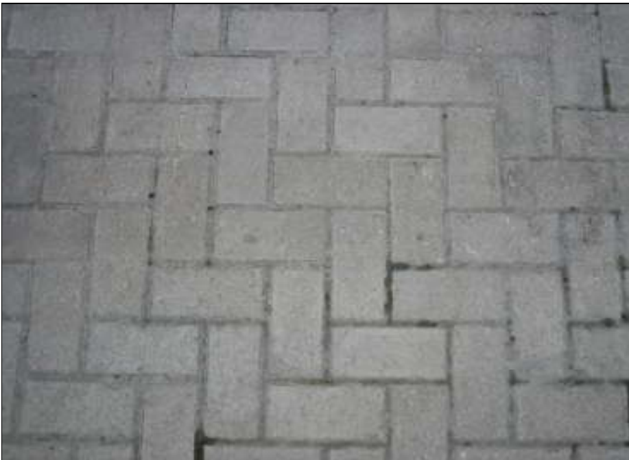
Photograph 2: Demonstrating intact nature of hardstanding
