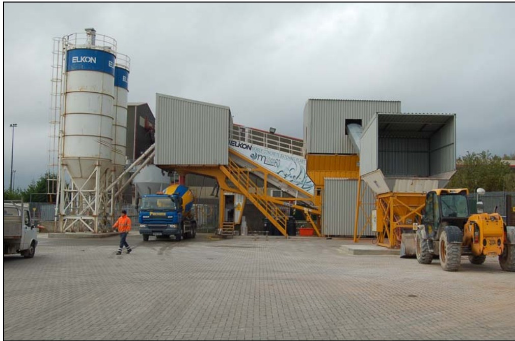
Photograph 2: The Llay Plant in Operation (view east to west)
