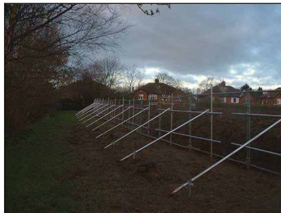
Actual barrier being erected on site – incorporating Heras type panels
