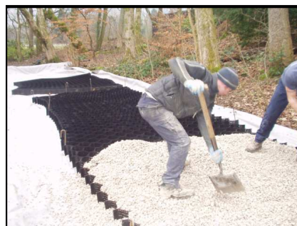
Photo 3- expanding and filling the Cellweb system
