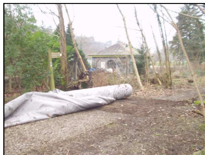
Photo 2- laying of Fibretex material onto existing subgrade
