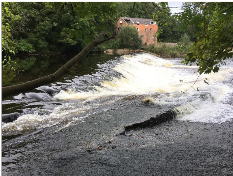
Figure 13: Erbistock Weir – concrete ramp and baulk fish pass
