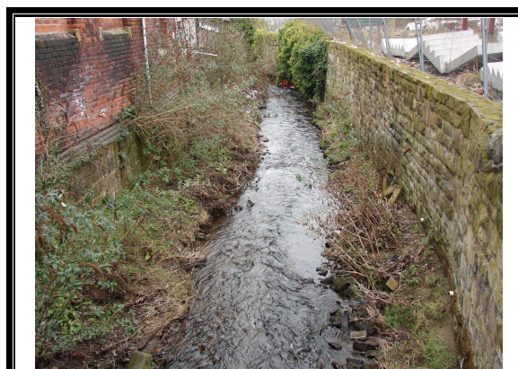
River Gwenfro from Willow Bridge on Salop Road. Survey site is to the right of this view.
