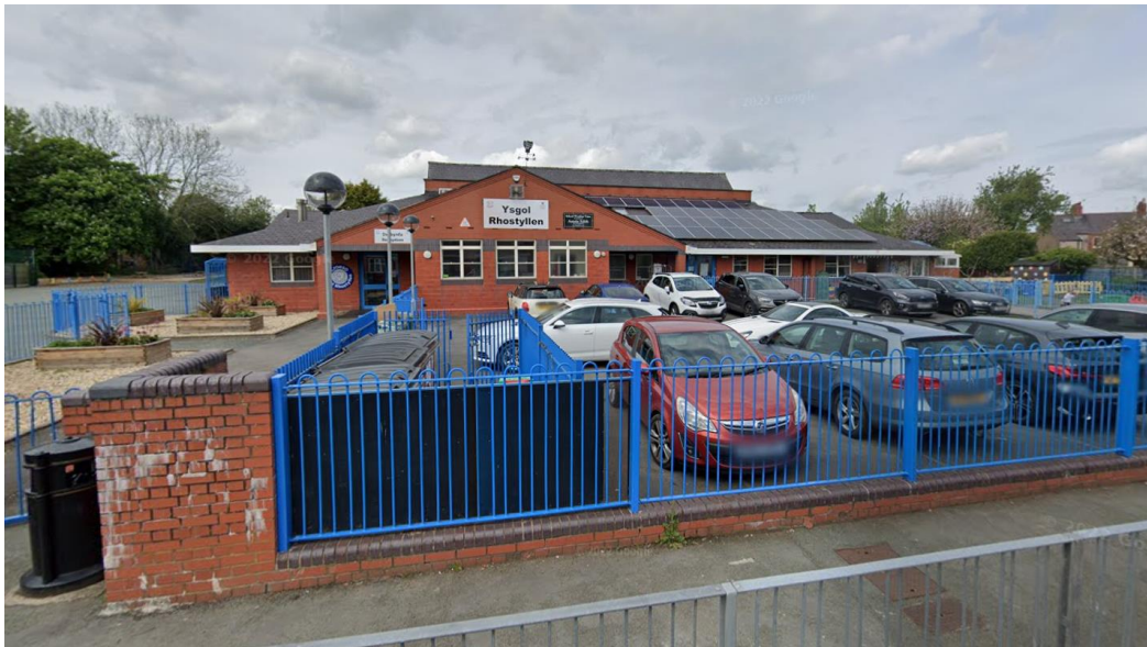
Existing classroom building with cement fibre horizontal boards
