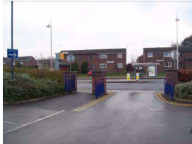
Entrance Mold Road
