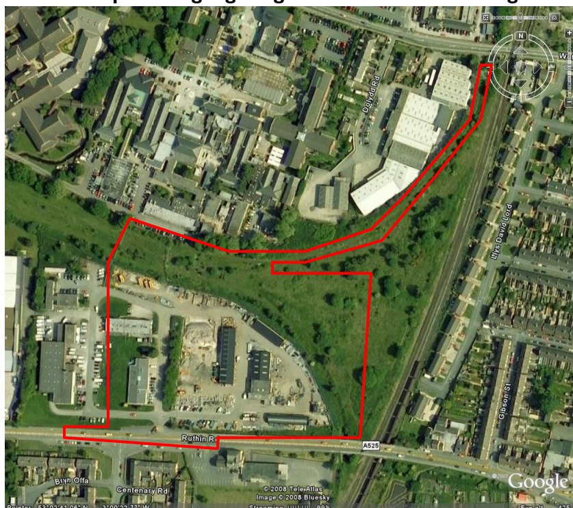
Figure 01 Aerial photo highlighting the site and surrounding land uses
