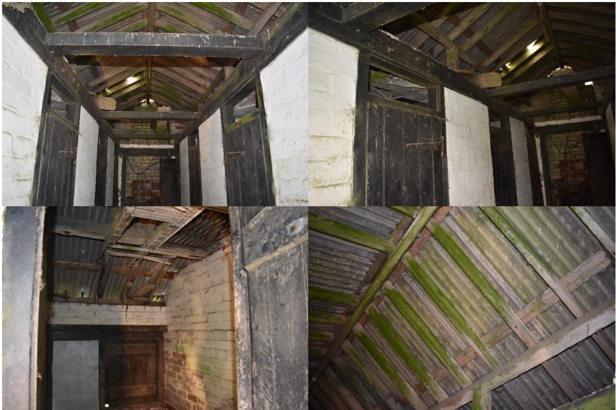
Figure 3.10: The interior of the kennels building.
