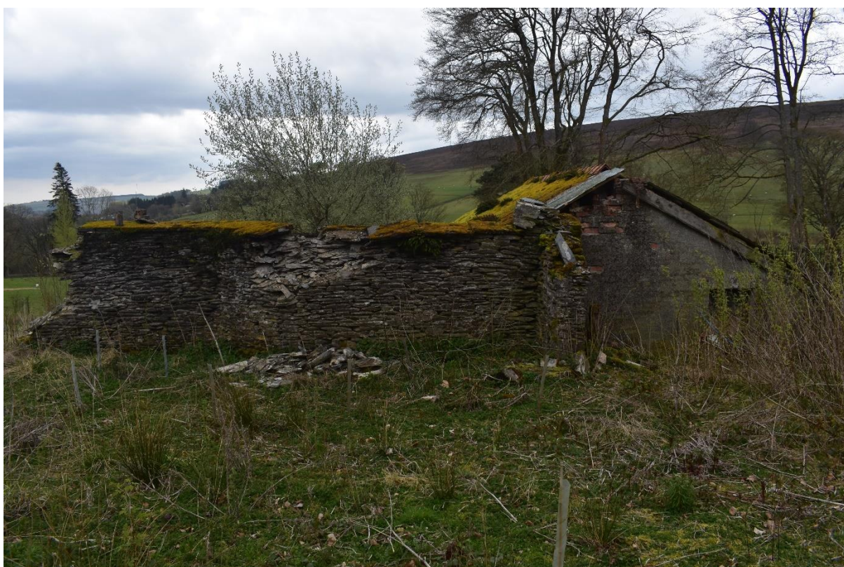
Figure 3.4: The rear (northwest-facing) elevation of the kennels building. The stone wall which adjoins the rear of the building can be seen on the left of the image.
