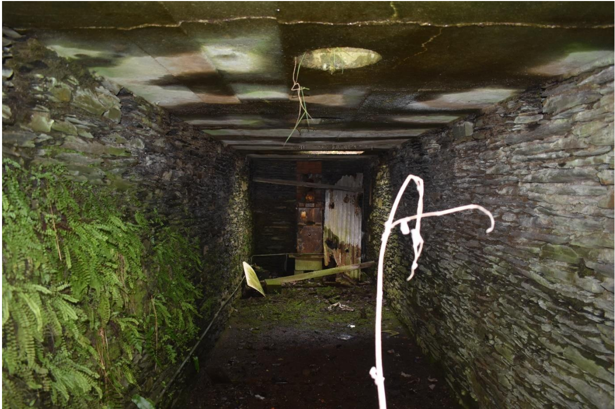
Figure 3.11: The subterranean boiler room.
