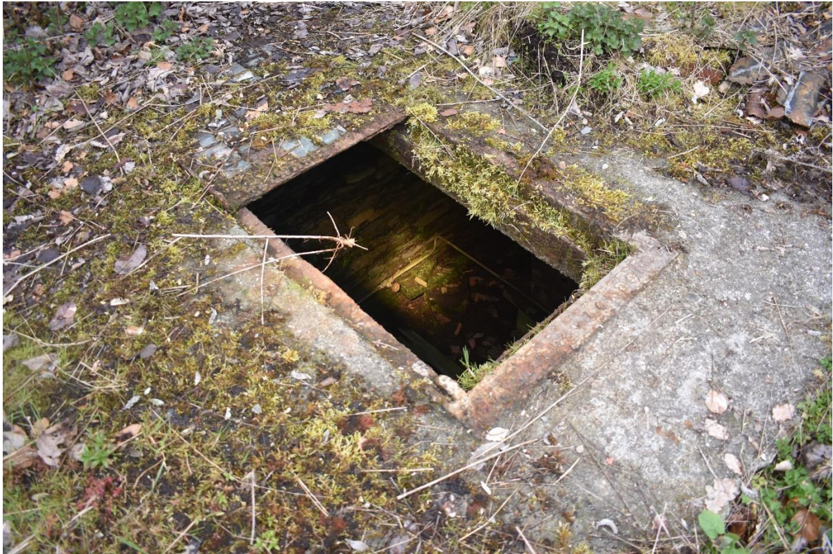
Figure 3.13: The top access to the boiler room.
