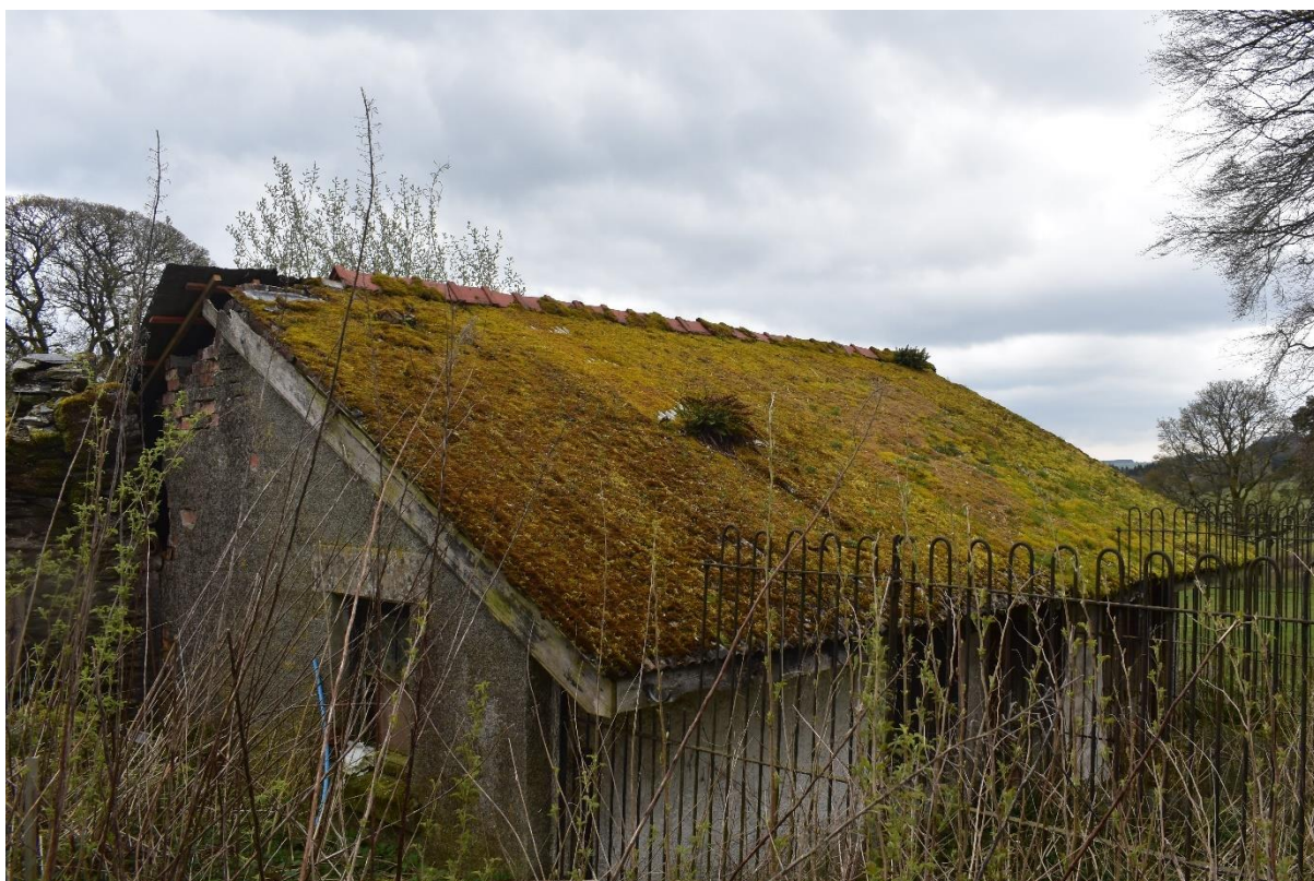
Figure 3.5: The roof of the kennels building.
