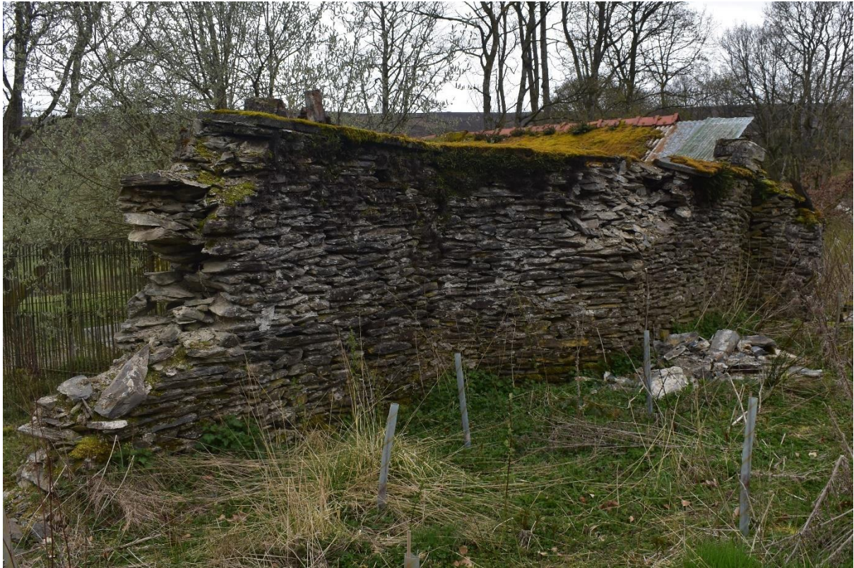
Figure 3.9: The stone wall which adjoins the rear of the kennels building.
