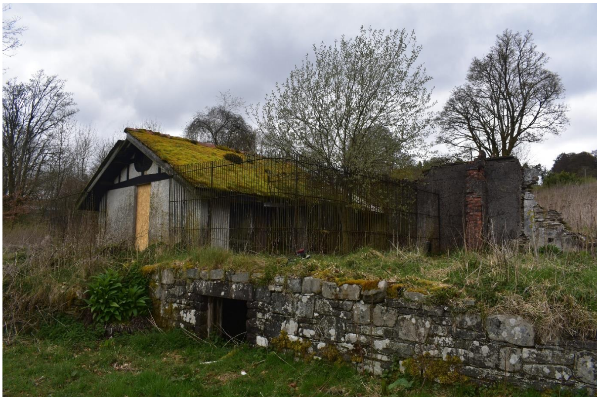
Figure 3.2: The front (southeast-facing) and northeast-facing side elevations of the kennels building. The roadside access to the boiler room can be seen in the foreground.
