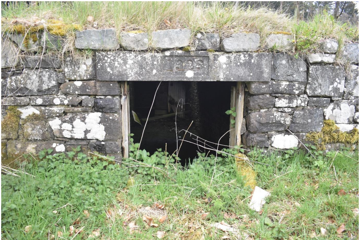
Figure 3.12: The roadside access to the boiler room.
