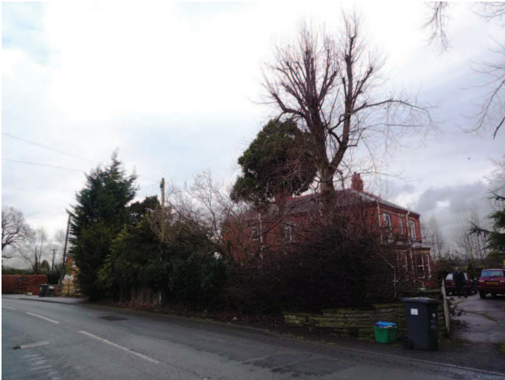
Photo 2 – Site frontage viewed from west – note poor past management & unkempt appearance
