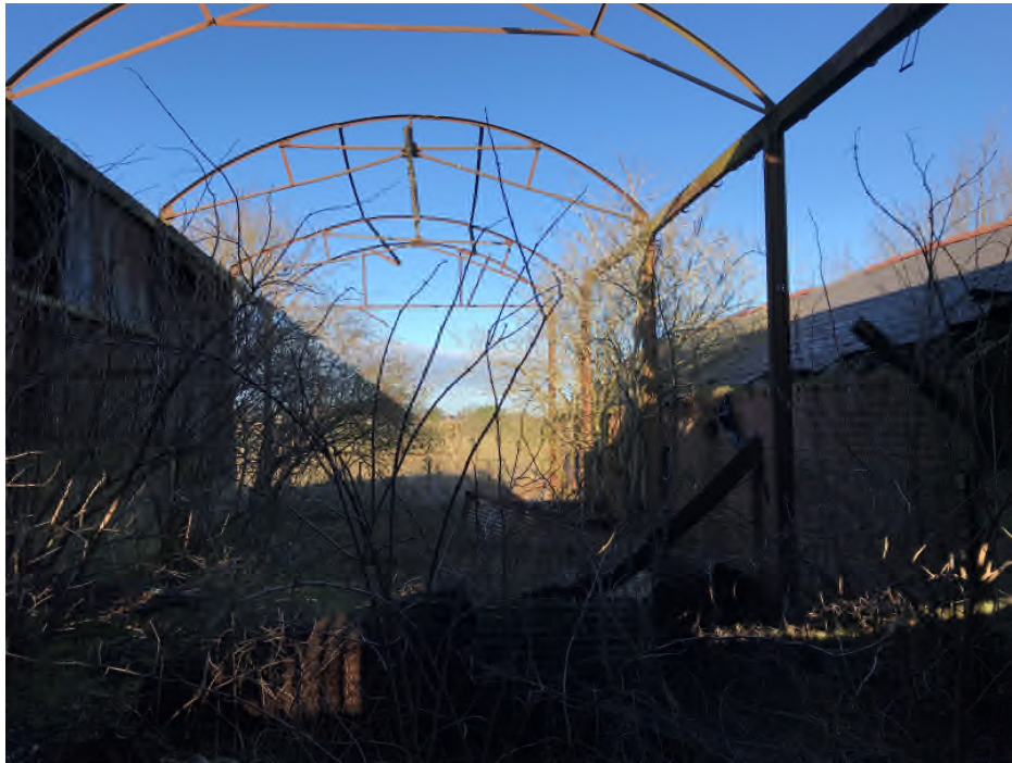
Building 3 view through structure
