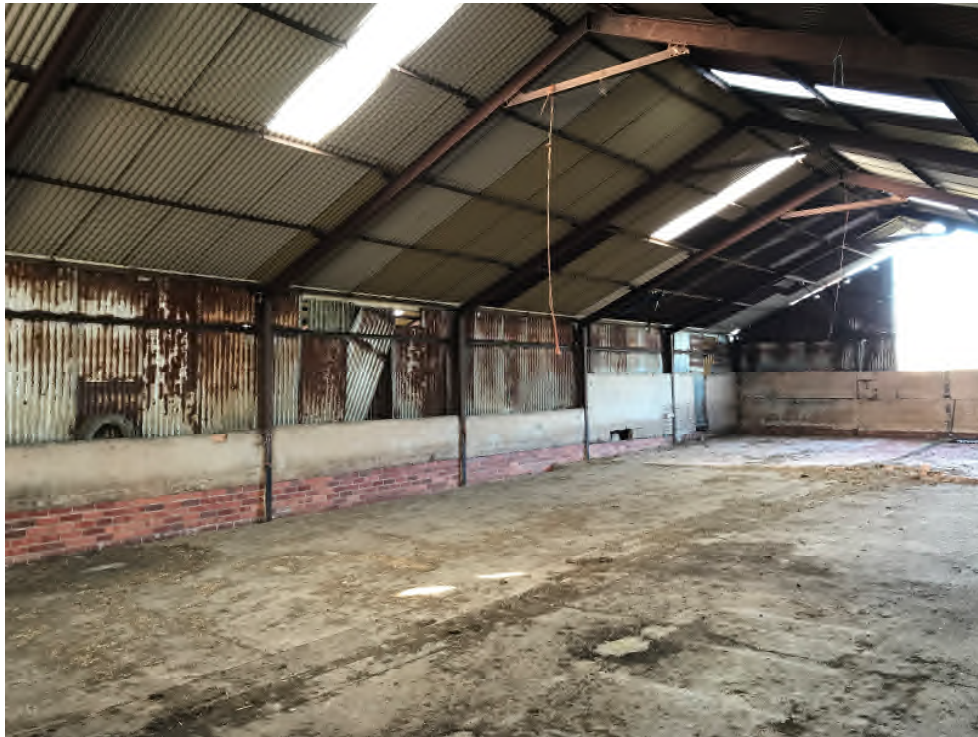
Building 9 view through structure
