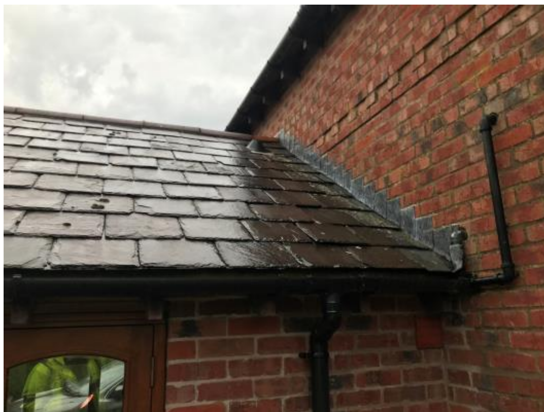
Plate 2 – Character of the slate roof
