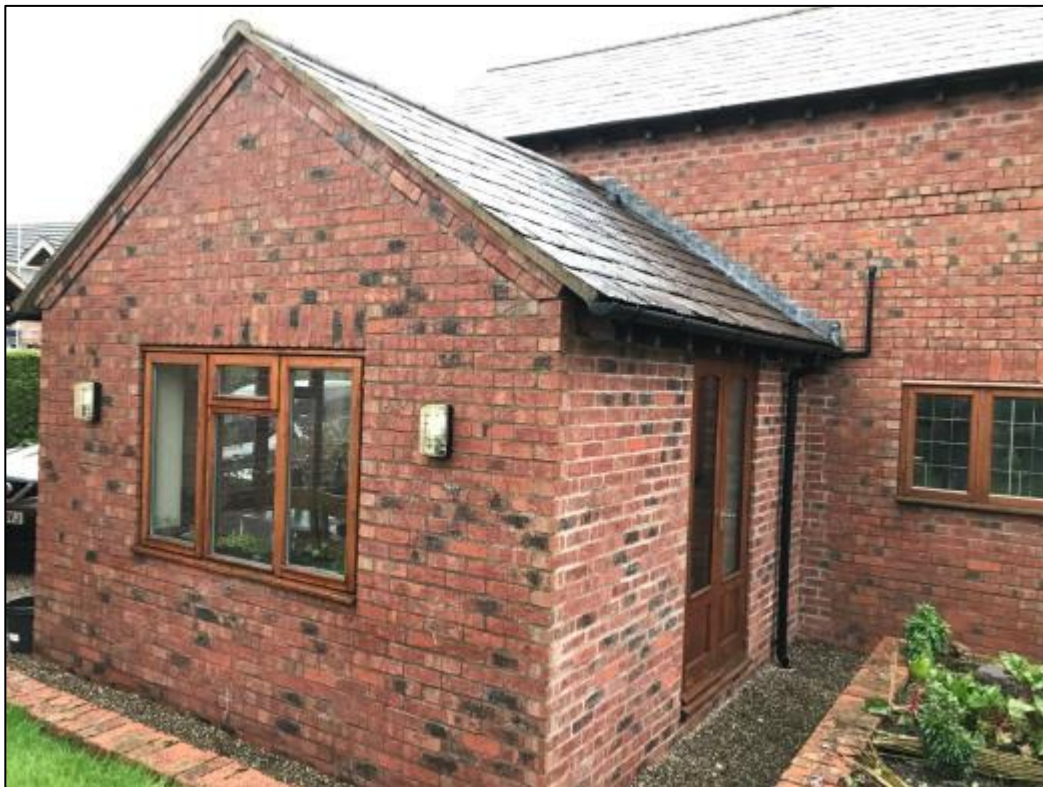
Figure 7.1 – The existing extension to be demolished, with the two-storey section to be retained behind.
