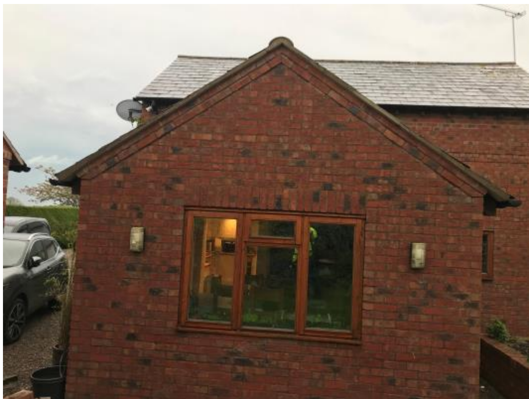
Plate 1 – The existing single-storey extension viewed from the north
