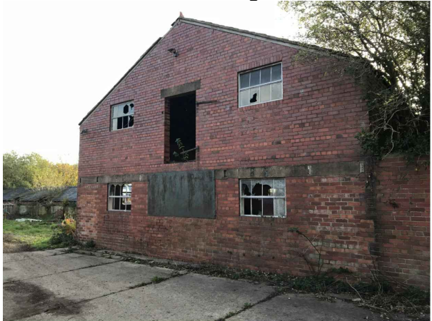
Rear elevation of building 15
