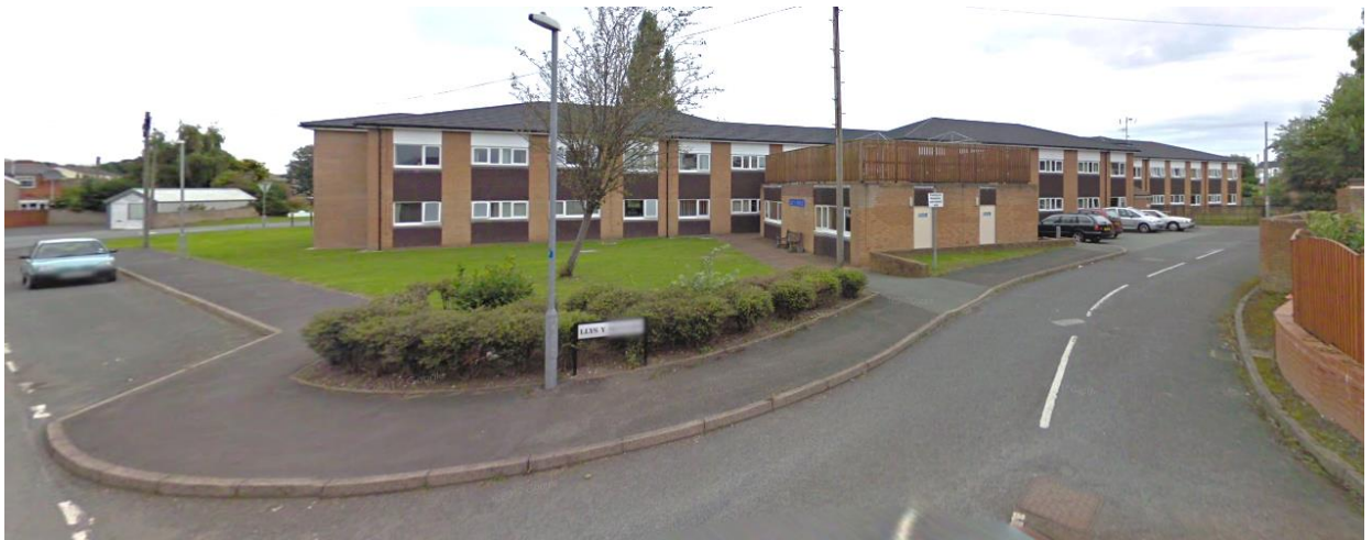
View from Llŷ y Mynydd entrance (south elevation)
