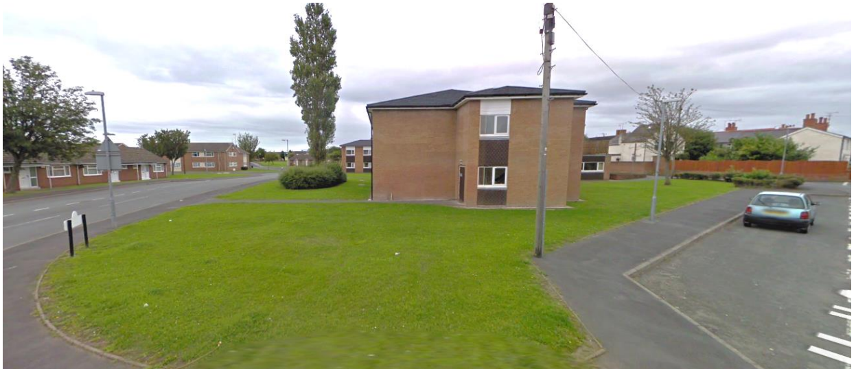
View from Hall Street (west elevation)
