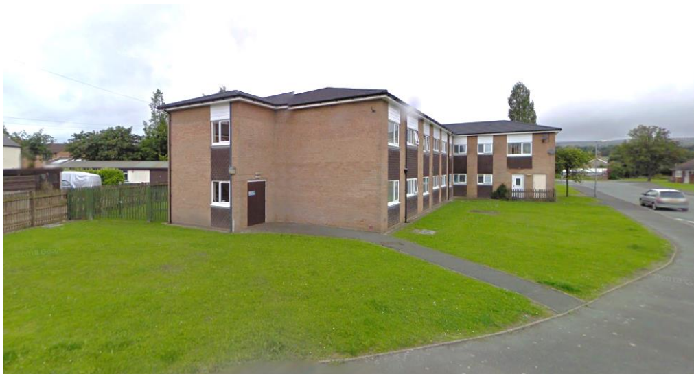
View from Campbell Street (east elevation)
