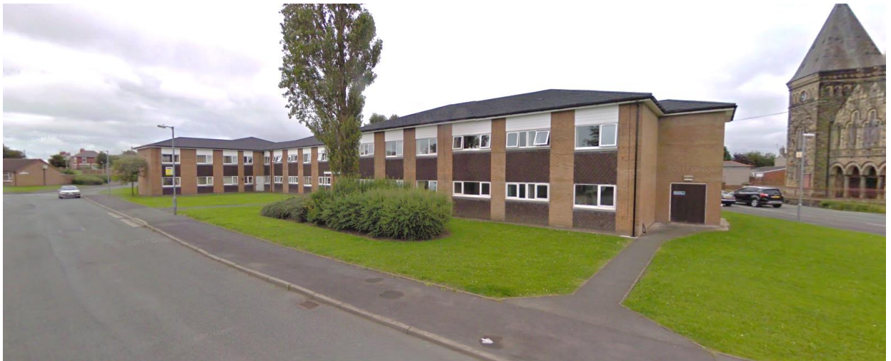
View from Mountain Street (north elevation)
