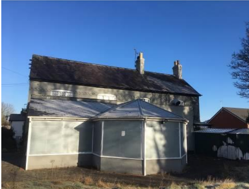
Plate 3: Southern elevation of B1
