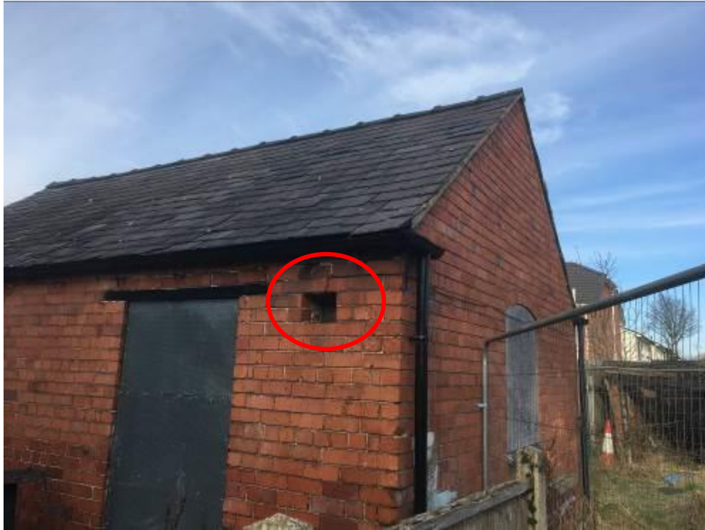
Plate 11: External character of the outbuilding B1 from the south-east, with a gap leading into the interior
