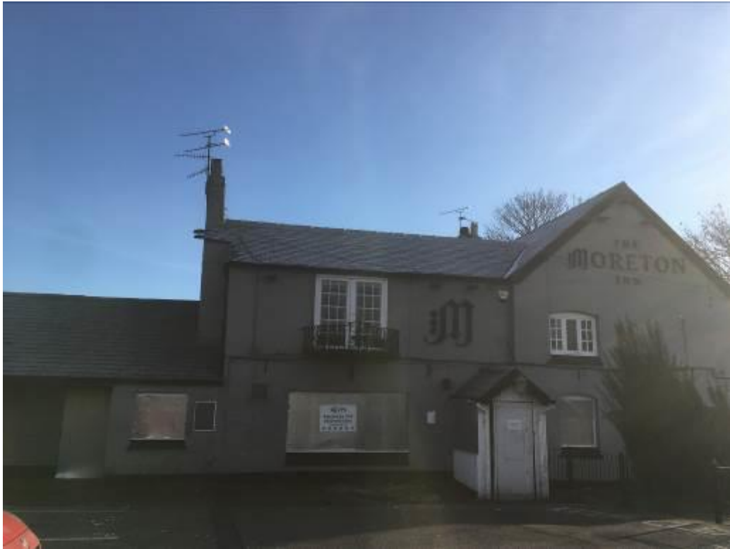
Plate 1: Front (western) elevation of the former Moreton Inn
