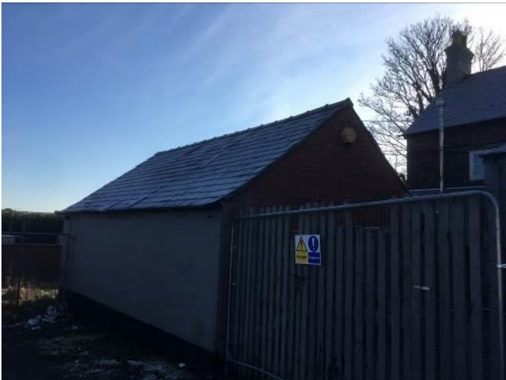
Plate 10: External character of the outbuilding B2 from the north-west
