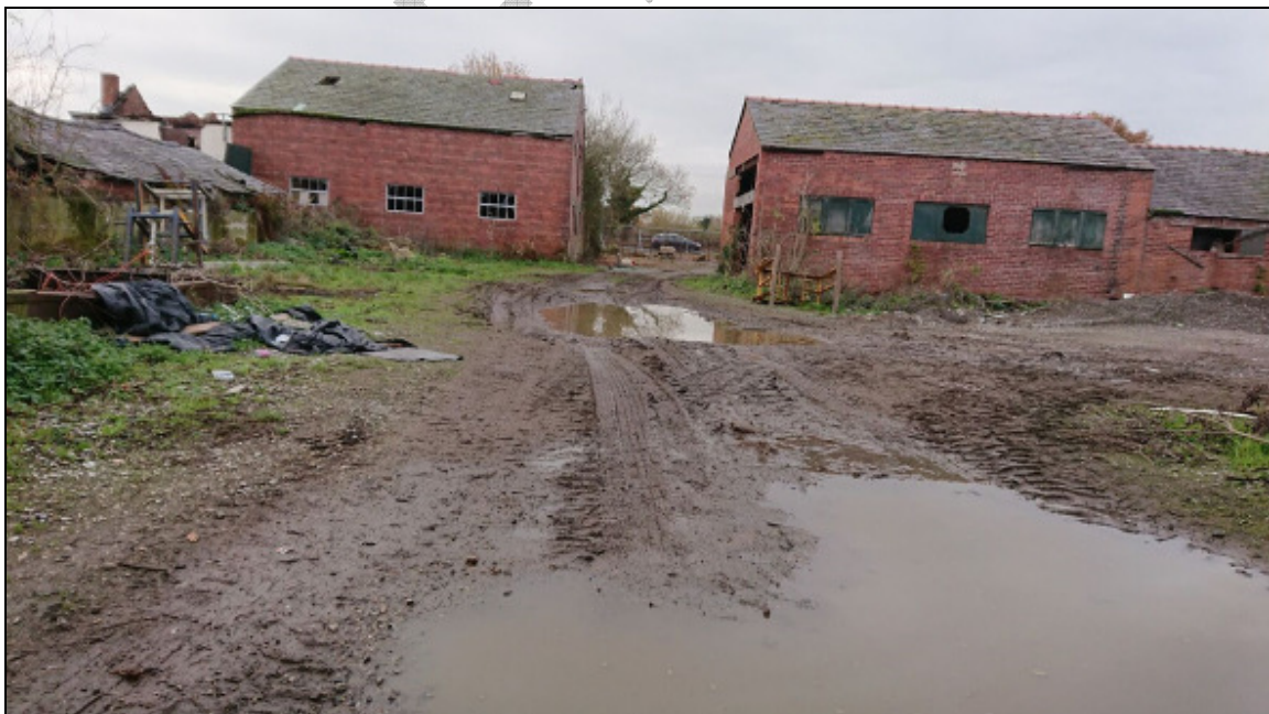
Plate 8 - Image taken from the centre of the site looking south, you can see Buildings 3 (red brick centre left) and 6 (red brick, centre right)
