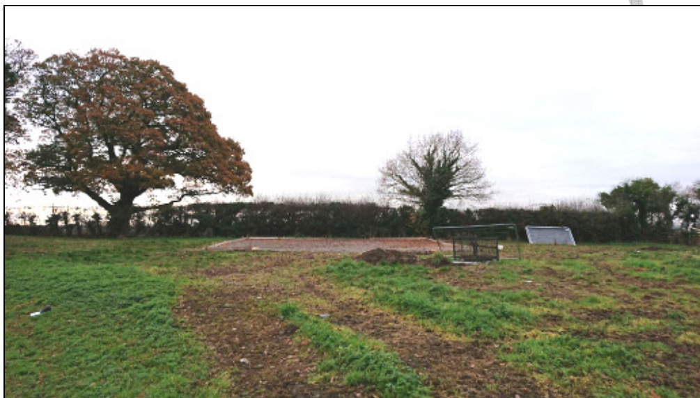
Plate 10 - Newly built building foundation, Target Note 5
