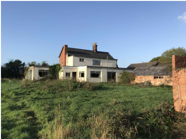
Rear elevation of building 20
