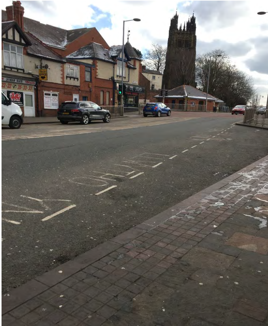
Existing loading bay adjacent to site on Brook Street
