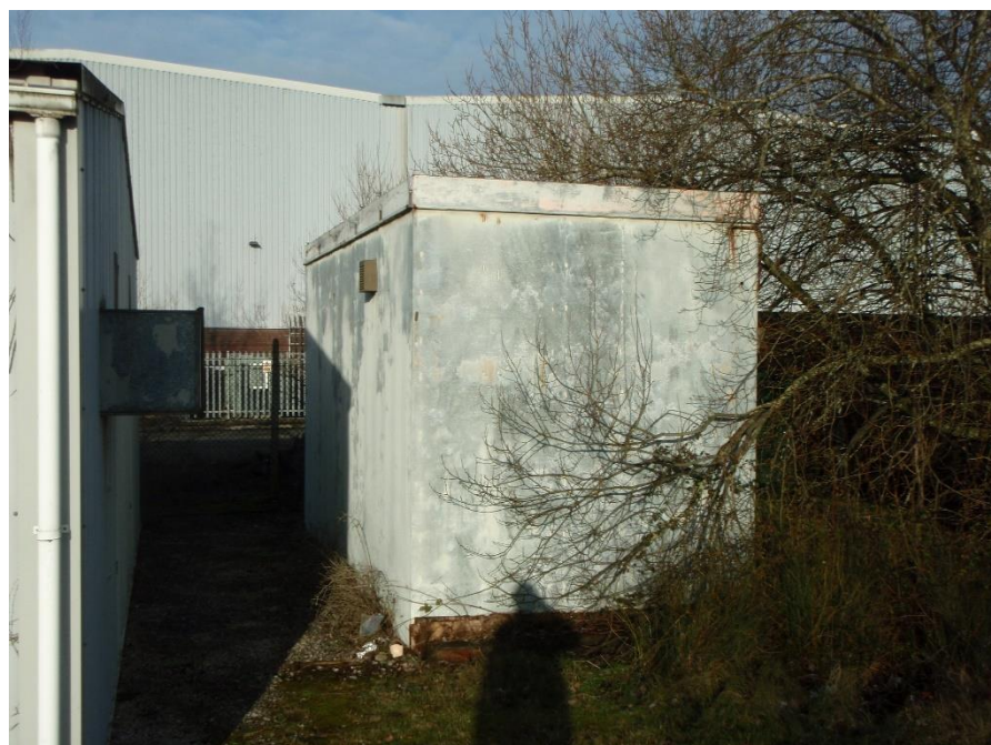
Structure at Target Note 1d . Photo taken 01/02/21.
