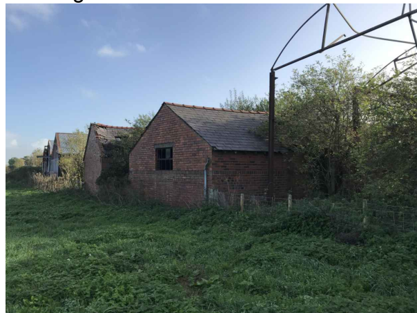
Side elevation of building 4 & 5
