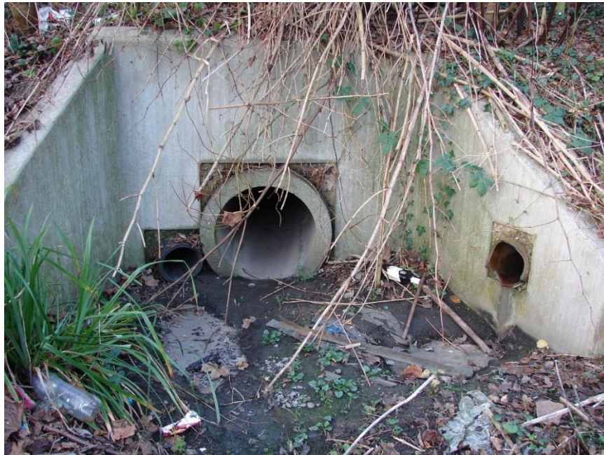
Drainage pipe at Target Note 1 .
