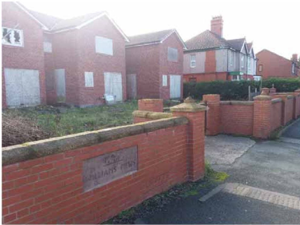
Photograph 1 Site from Ruabon High Street, prior to demolition
