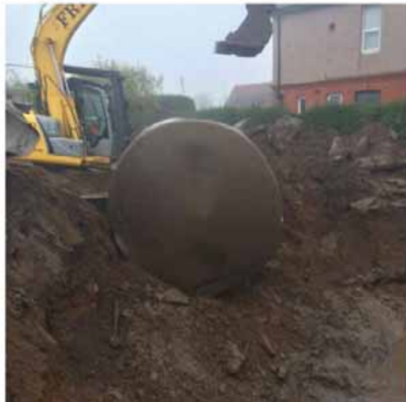
Photograph 2 – Tank being removed from excavation
