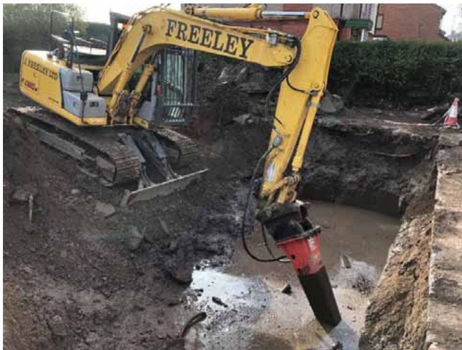
Photograph 3 – Breaking out underlying concrete slab.
