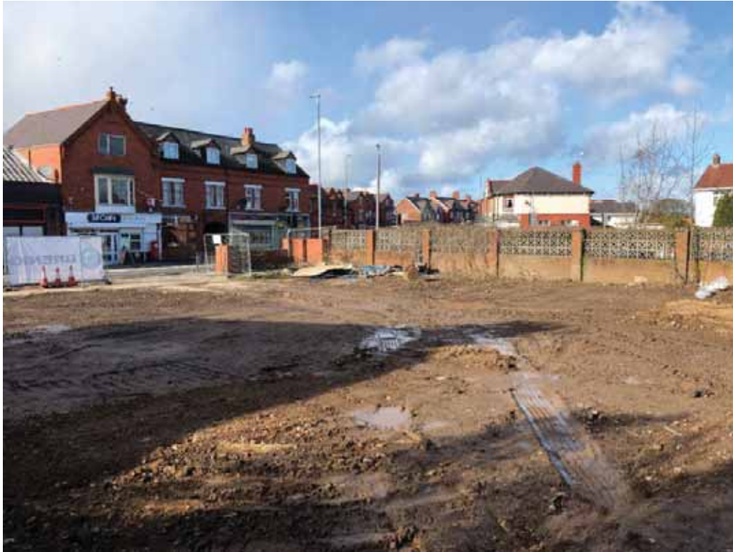
Photograph 5 Site area following demolition of buildings
