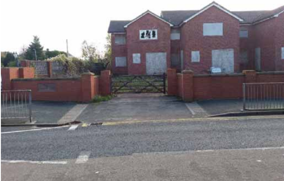
Photograph 2 Site Entrance, prior to demolition
