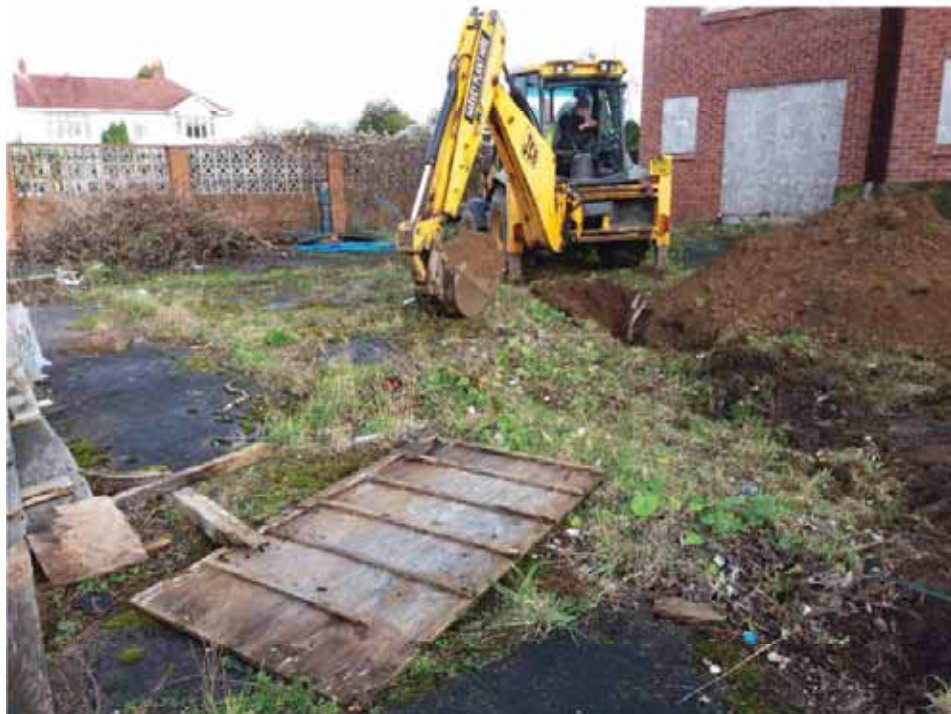
Photograph 4 Concrete and tarmac hardstanding in western part of site, prior to demolition
