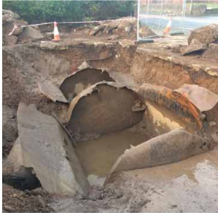
Photograph 1 – Tank (internally divided into two) prior to removal
