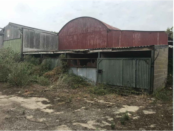
Rear elevation of building 3
