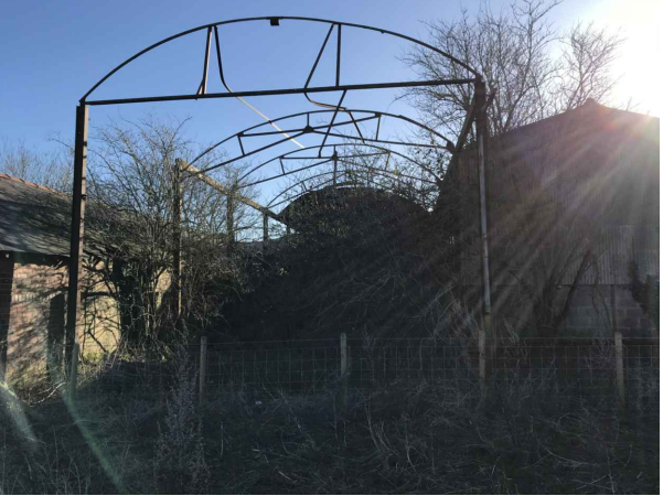
Front elevation of building 3
