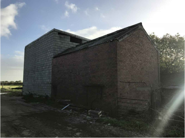
Side elevation of building 10
