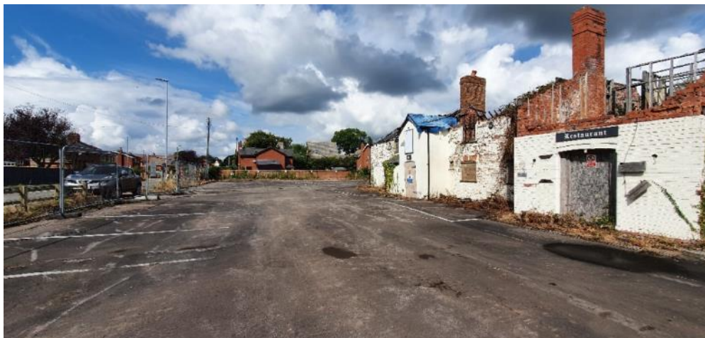
Site facing north west
