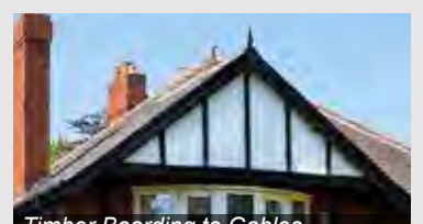
Timber Boarding to Gables
