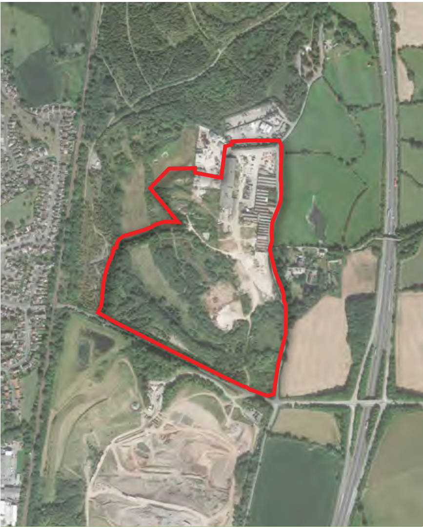
Aerial view of the site, with application site boundary edged in red.
