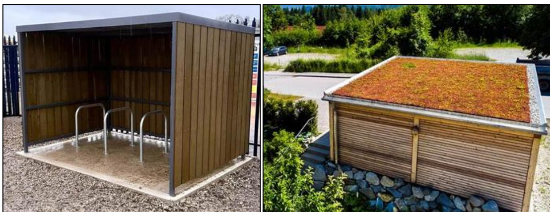
Figure 6.1 – Left: covered bicycle storage area, and right: example of a building with sedum roof.
