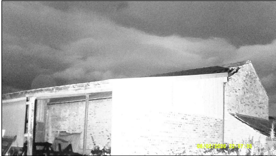
Figure 3.1 – NVA image of B1, from dusk survey 1, as viewed from the north-west
