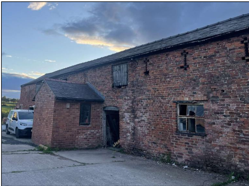
Figure 4.1 – Character of the southern elevation of B1
