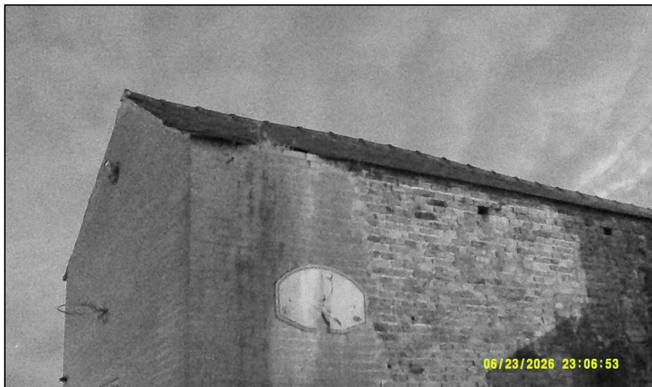
Figure 3.2 – NVA image of B1, from dusk survey 2, as viewed from the north-east
