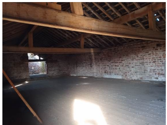
Photos 16 and 17 – General views of first floor store.
