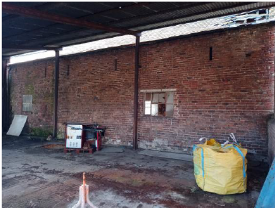
Photos 7 and 8 – Rear Elevation.
