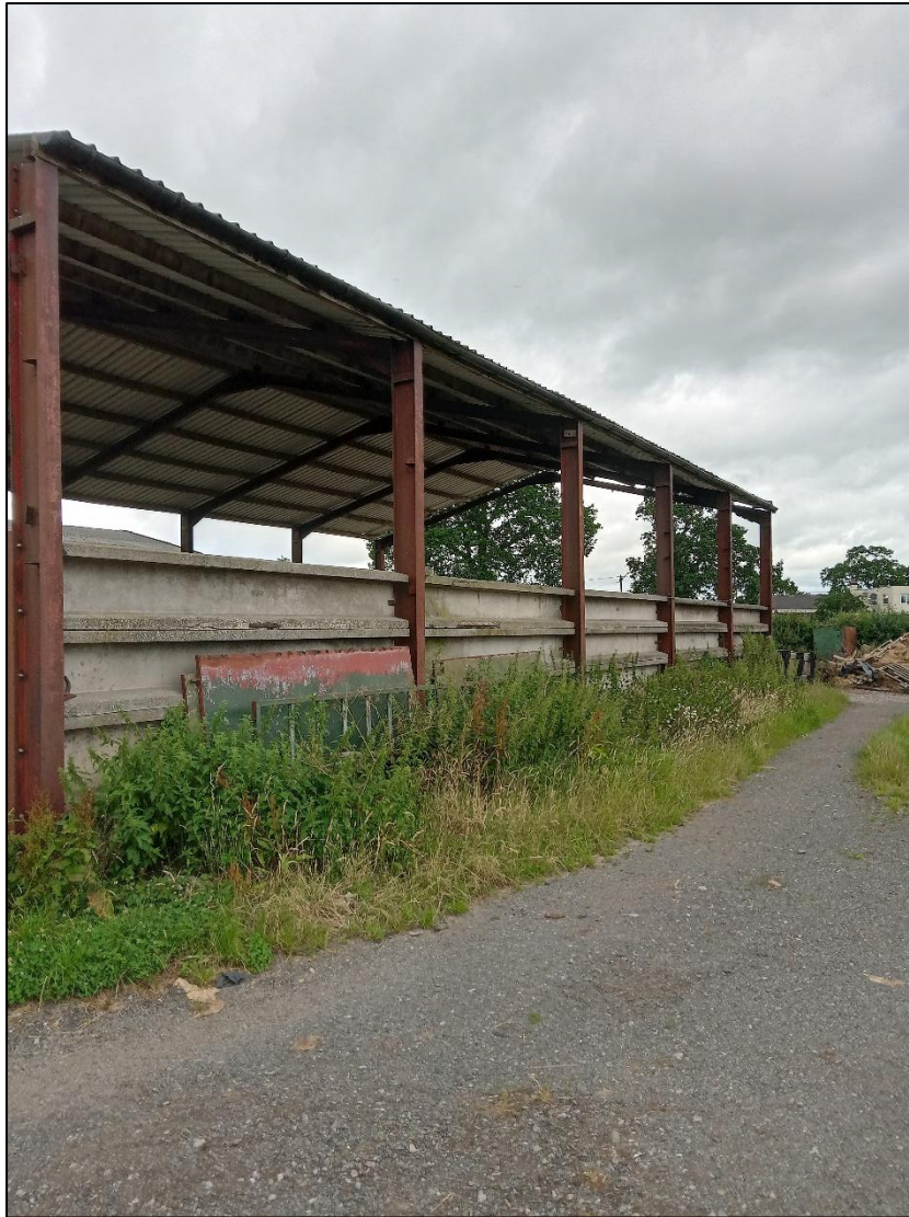
Figure 6: Building B viewed from the east
