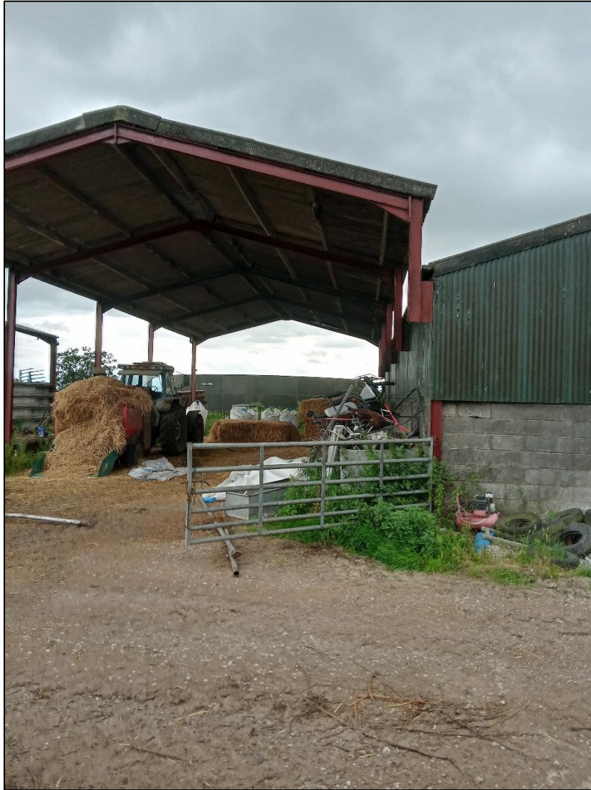
Figure 7: Building D viewed from the north
