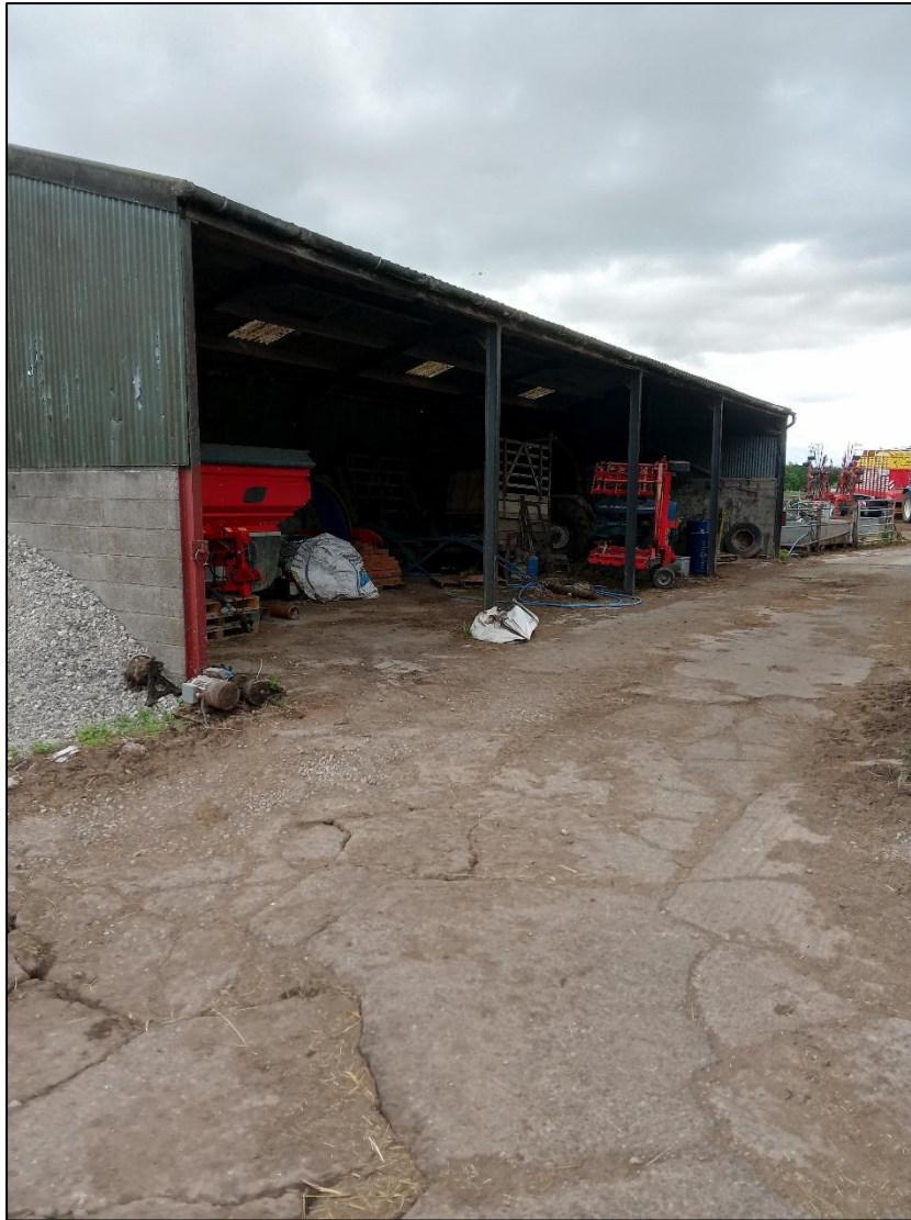
Figure 8: Building E viewed from the north-west
