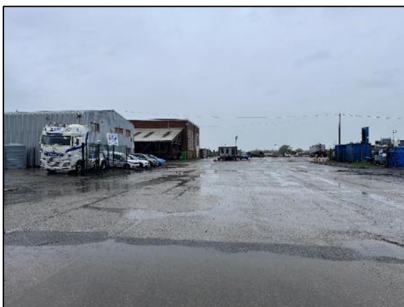
Figure 11: Buildings that may provide roosting opportunities.
